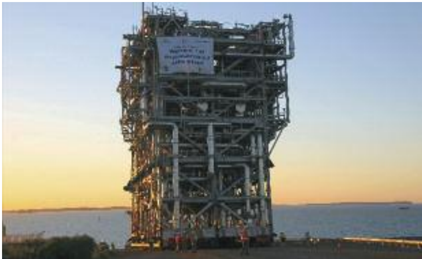
Figure 1.1 - One of the pre-assembled units for the Woodside-operated Train V Phase 5 LNG expansion facility at Karratha, Western Australia.
