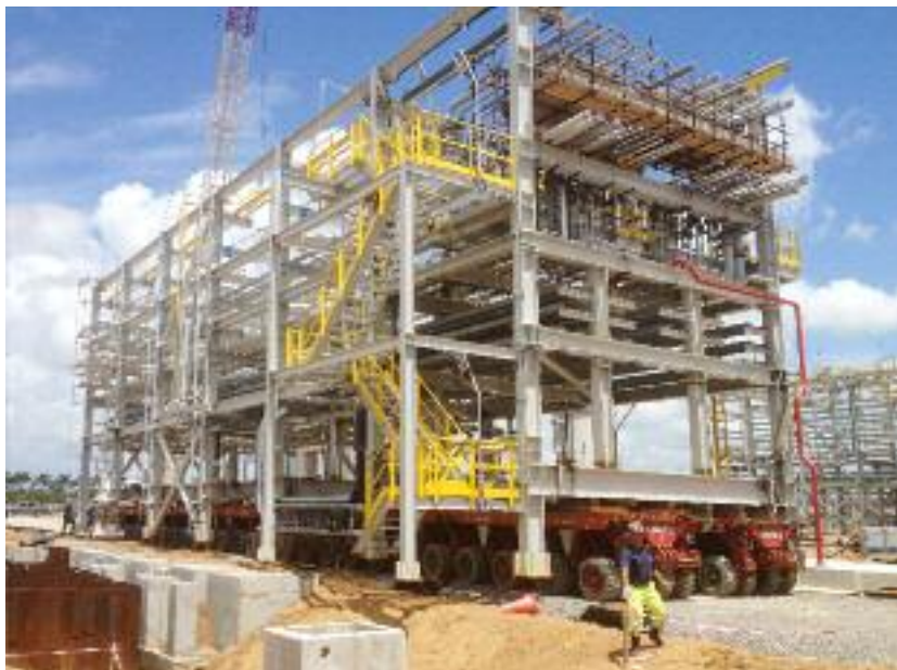
Figure 1.4 - Installation at site of a module fabricated by Saipem at Arbatax yard for a refinery in Suriname (By Fagioli)
