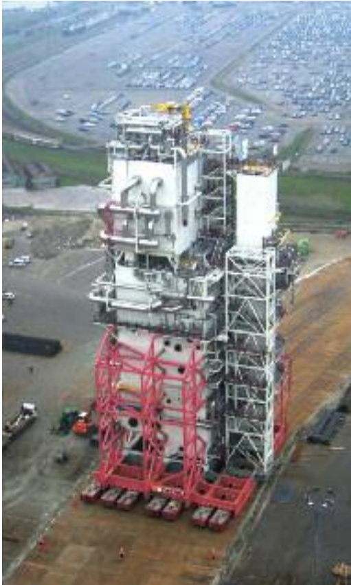
Figure 1.12 - A modularised cold box for an LNG plant at Hammerfest, Norway . The unit, that had a weight of 2700 tons and was 60 meters high, was transported from Belgium to Norway by barge and then a semi-submersible ship. (By Fagioli)
