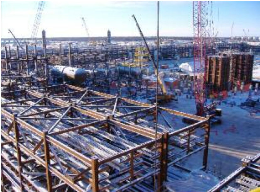
Figure 1.6 - A view of the Horizon Oil Sands Plant, Fort Mc Murray, Northern Alberta, Canada. In the last decades modularization has been largely adopted in order to mitigate the impact of severe weather conditions at site (By Technip)
