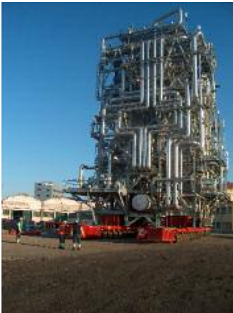
Figure 1.2 - Modularized steam reformer furnace for hydrogen production unit, designed and built by Foster Wheeler for a plant in Nigeria.
