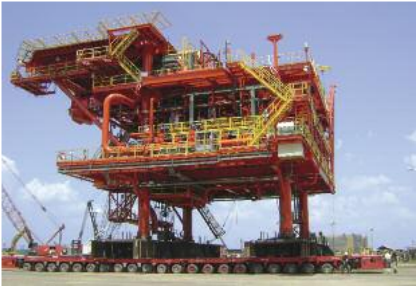
Figure 2.3 - The 25 meters deck of an offshore plant on a Self-Propelled Modular Trailer (By Fagioli)
