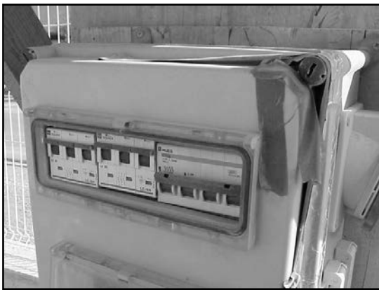
Figure 2. Example of non-satisfactory maintenance level of an electric panel
