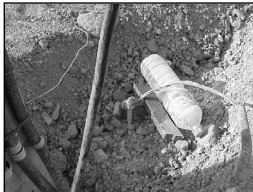
Figure 7. Grounding connection not protected
