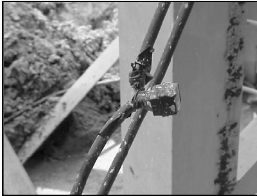
Figure 5. Broken cable with a "temporary" union
