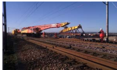
Deck Construction and S&C Installation
